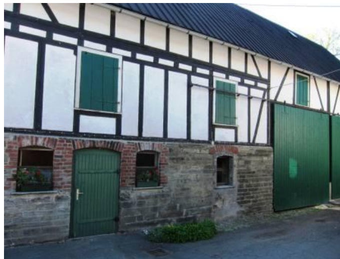
Front side of Abraham of Balde’s barn called “Wahnersch”. The barn has been extensively enlarged and renovated.
