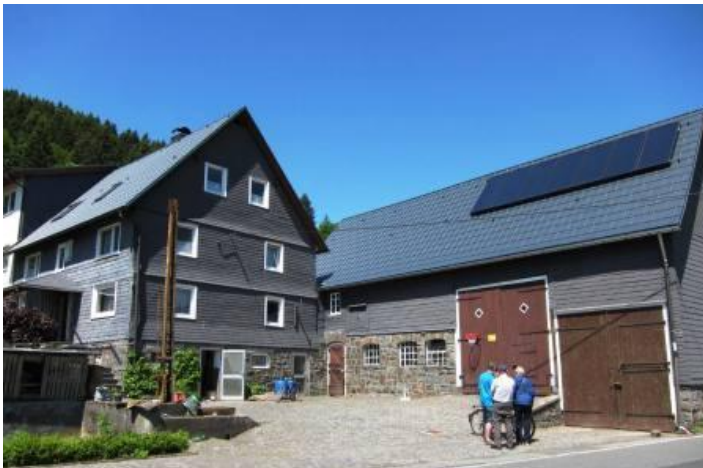
The house in Steinbach called "Jost's" belonged to Simon's Grandfather, Daniel Treisbach about 1650. Since then it has been greatly enlarged and the half-timbers covered with slate.
